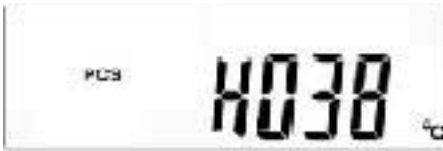
Fig. 7-4 - 3 Display I - Temperature of cooling element in °C
